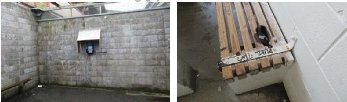
Figure 3. Examples of moss on walls and graffiti in the high security facility exercise yards
