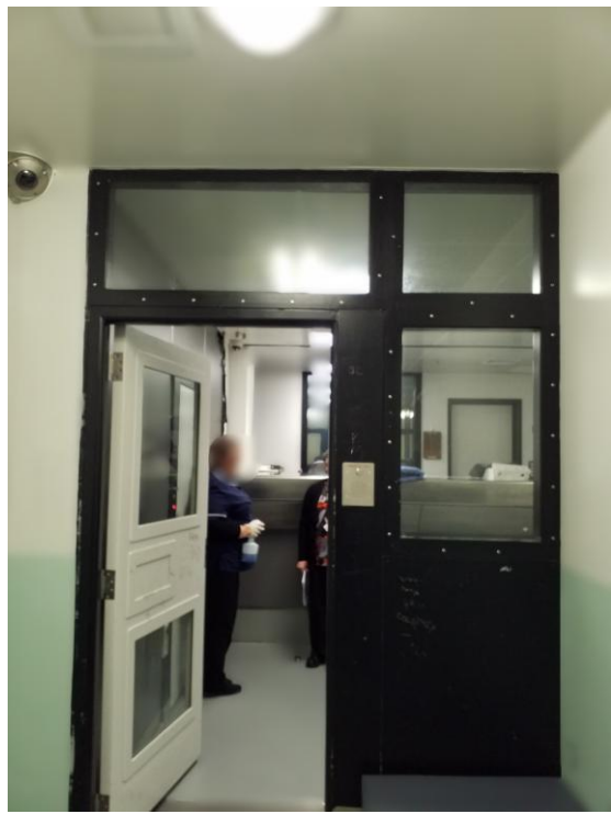
Image 20: View from inside the New Plymouth Remand Centre at-risk cell
