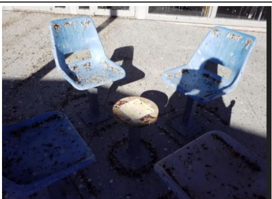
Photo 14: The outdoor courtyard of the main visits area was closed due to the pigeon infestation.
