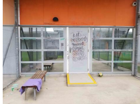
Image 2. Auckland Region Women's Corrections Facility Management Unit yard.
