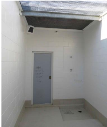
Image 7. Christchurch Men's Prison Kotuku Unit Separates yard.
