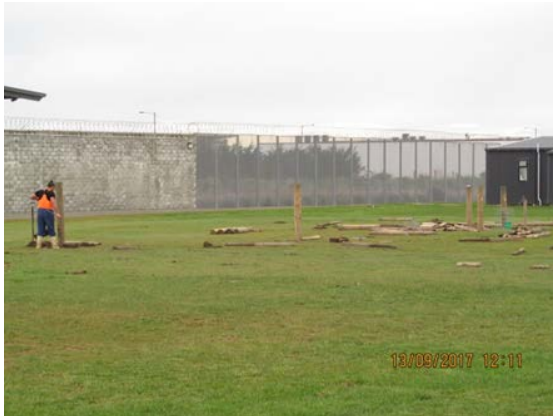
Fence building during agriculture course
