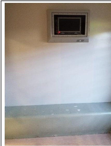
Image 1: Holding cell in the Receiving Office with concrete bench and television screen.
