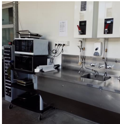
Image 10: kitchenette area in residential unit.
