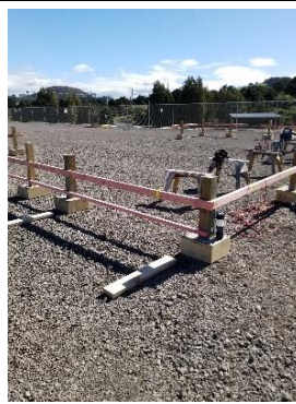
Image 18: Construction site at Innovation Park.
